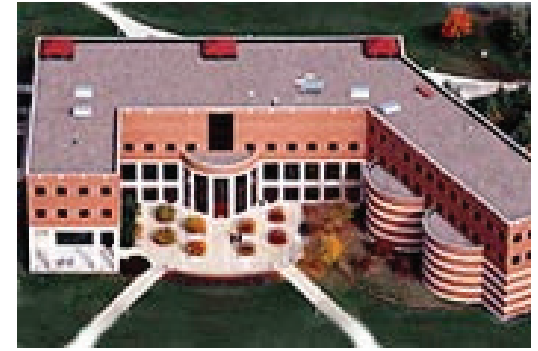
On the UNI campus in the Curris Business Building Room 28.
